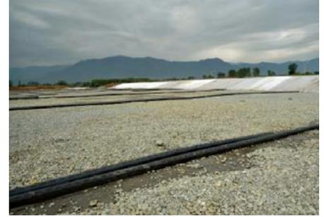
The underground drainage system for leachate collection
