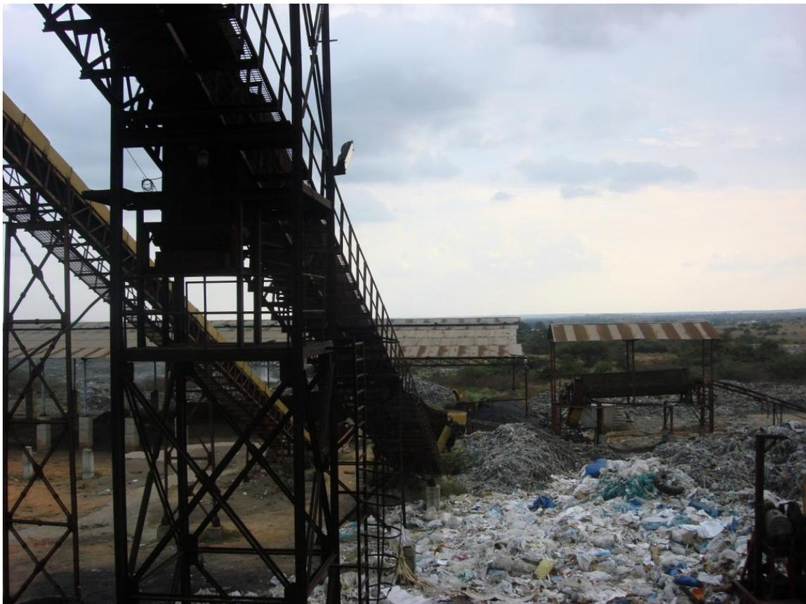
**Figure 34, Conveyor Belt for Feeding RDF into the WTE Boiler, Hyderabad RDF-WTE Plant, Elikatta**
